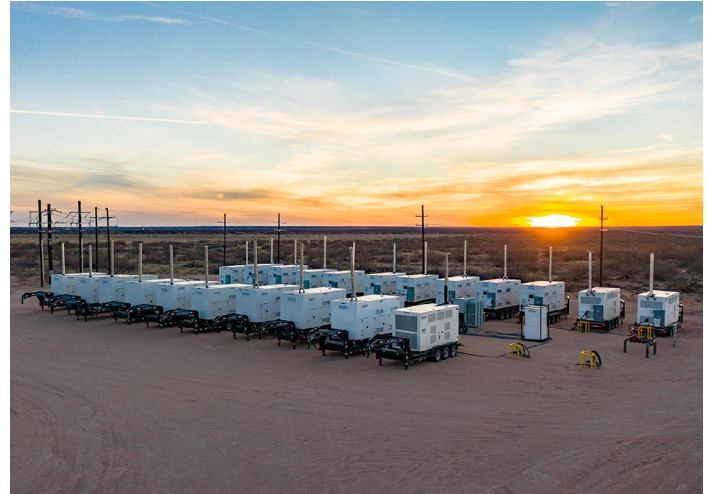
Baseline natural gas microgrid producing 8 MW (8,000 kW) of low-carbon electricity using in-field pipeline and produced gas.
